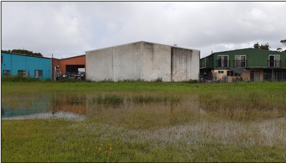
Figure 1: Typical site conditions facing southward near Bore 6.
